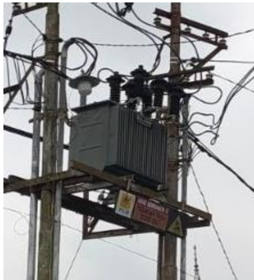
Gambar 2.2. Transformator Distribusi
