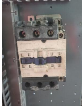
Gambar 2.5 Contactor
