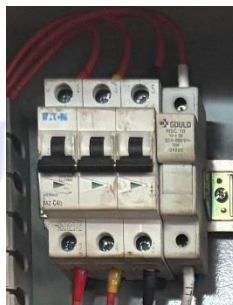
Gambar 2.1 MCB (Mini Circuit Breaker)
