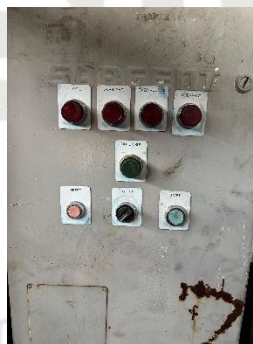
Gambar 2.10 Pilot Lamp
