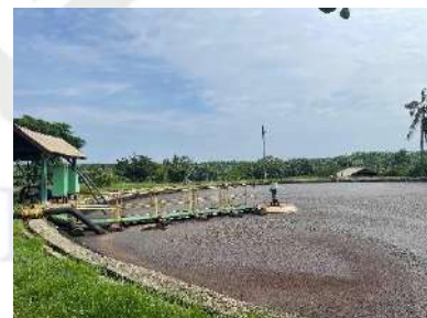
Anaerobic Pond
