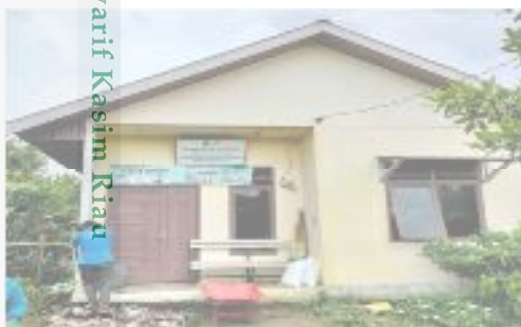
Figure 1 VCO Production Building
