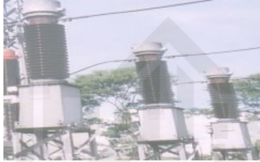
Gambar 2.10 Current Transformer (CT) [16].
