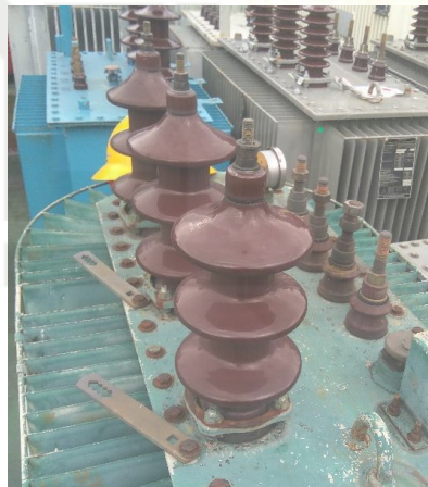
Gambar 2. 13 Bushing transformator[10]
