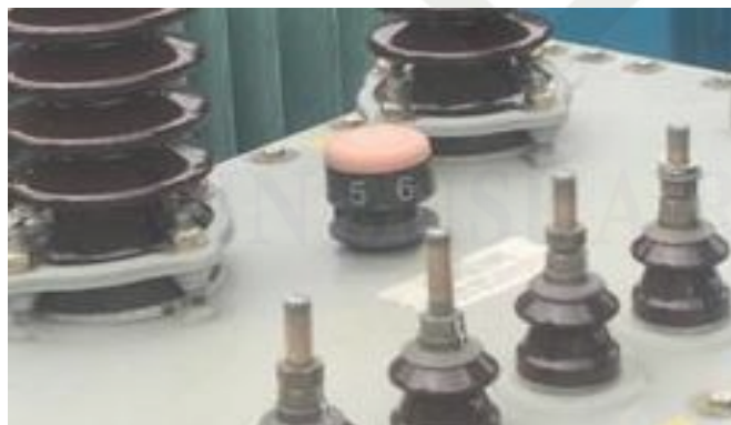
Gambar 2. 16Off load Tap Changer[10]
