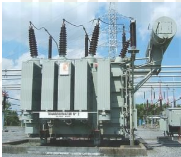
Gambar 2. 3 Transformator Step-Up [10]
