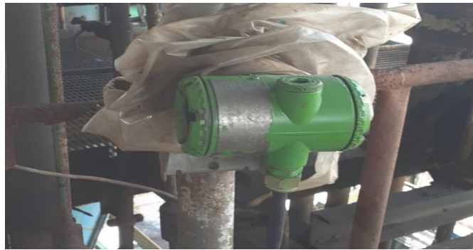
Gambar 2. 7 Differential Pressure Transmitter [14]
