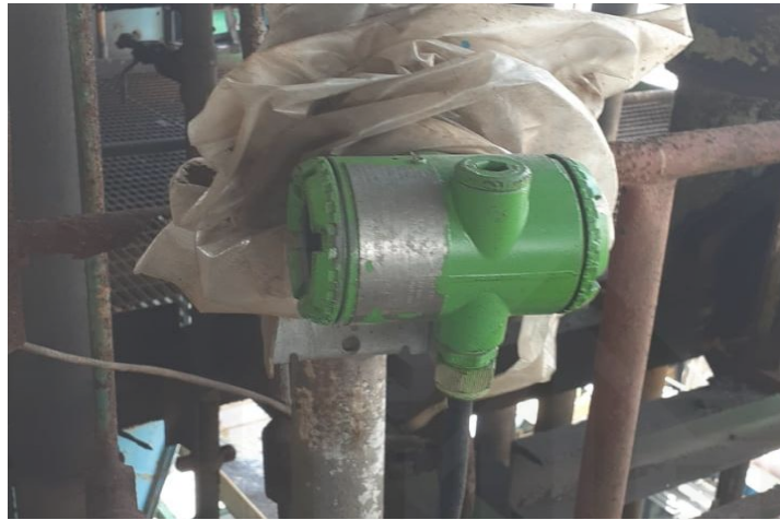
Gambar 2.7 Differential Pressure Transmitter [14]
