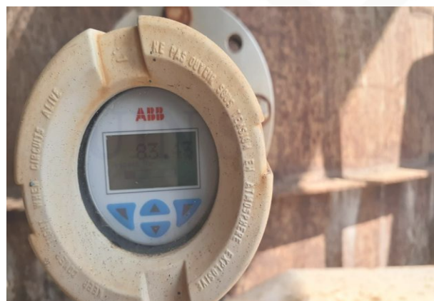
Gambar 2.6 Thermal Mass Flowmeter [14]
