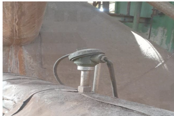
Gambar 2.5 Thermocouple PT100 [14]
