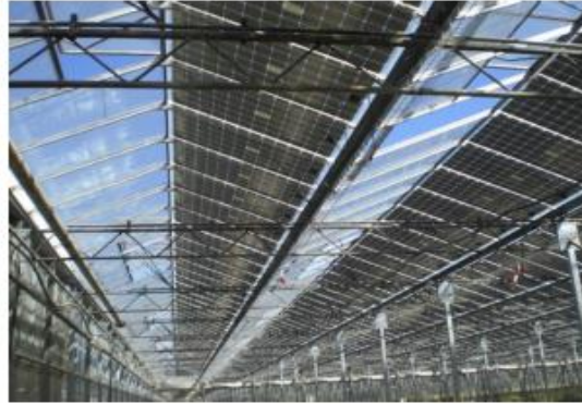
Gambar 2.16 STPV terintegrasi greenhouse [14]
