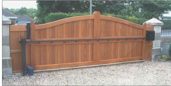
Gambar 2. 2 Pintu pagar geser ( sliding gate )
