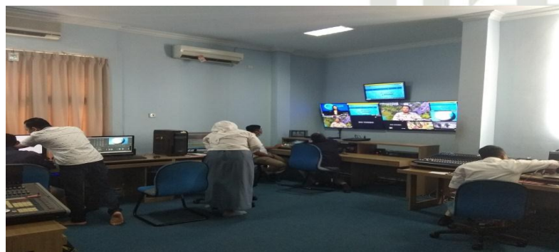
Gambar 5.2 MCR( Master Control Room). ( Doc. Peneliti )
