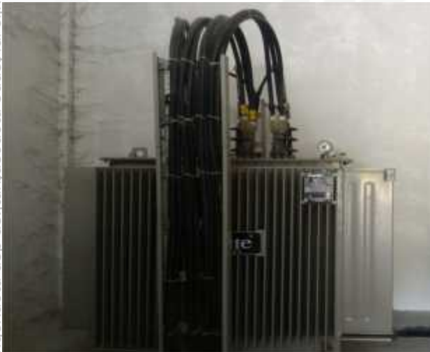
Gambar 3.1. Transformator distribusi 3 fasa
