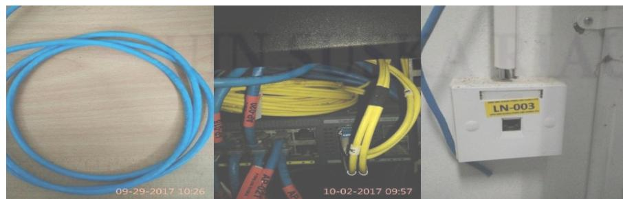
**Gambar 4.2 Kabel UTP (Kiri), Kabel FO (Tengah) dan Wall Jack (Kiri)**
